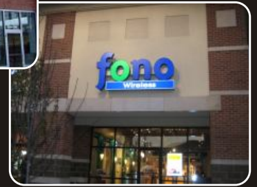
LED Illuminated Channel Letters, Mounted To A Raceway.
